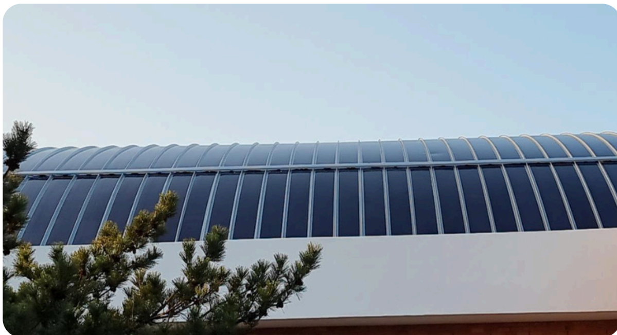
Roof of a gym_CIGS Flex32Kw
