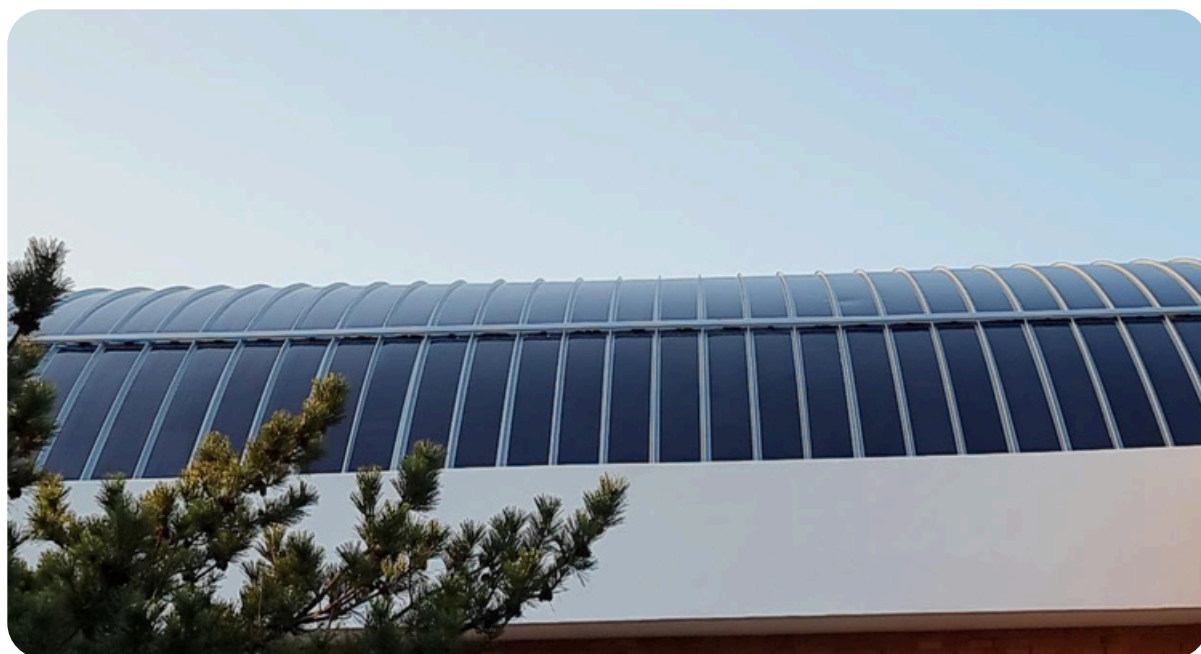
Roof of a gym_CIGS Flex32Kw
