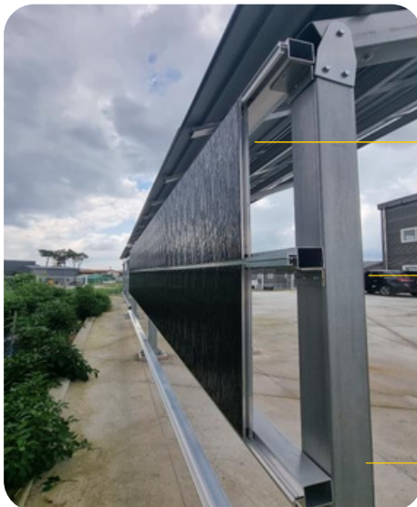
[Sash-type module frames and aluminum fixed studs]
