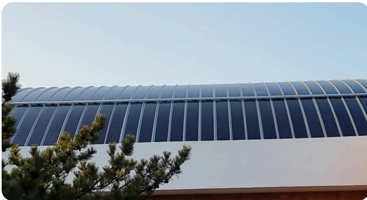
Roof of a gym_CIGS Flex32Kw
