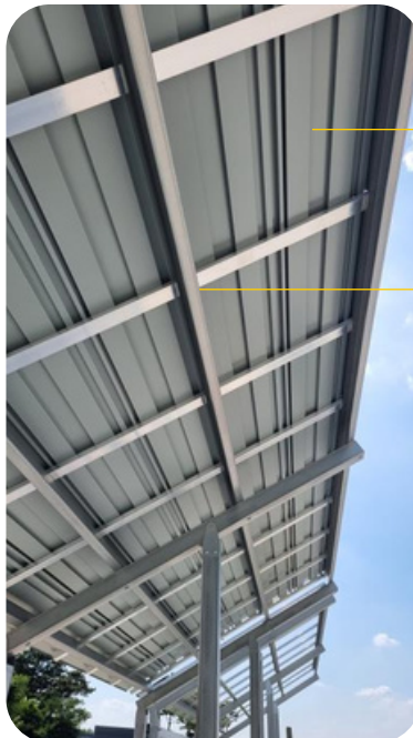
[Steel plate bending structure and PV module bonded together, aluminum fixed stud]
