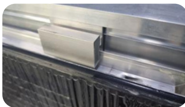
[Z-Bar module frame and clip fixed stud aluminum frame]
